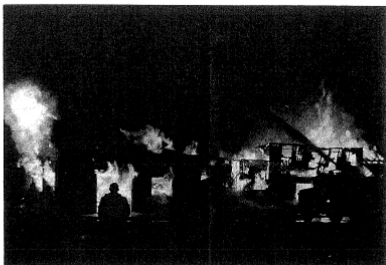
RAILROAD STATION FIRE - 1984
