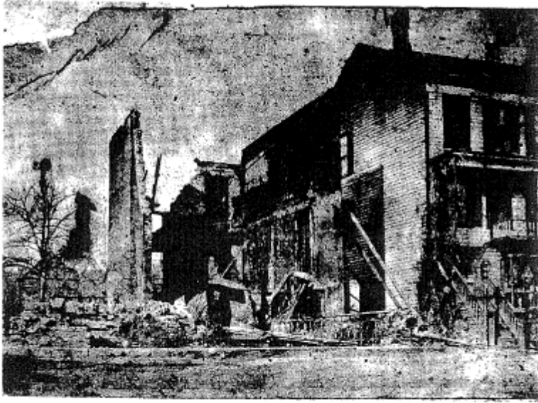
RUINS OF FERRIS BLOCK FIRE 1892, MAPLE BLVD. (FORMERLY R. R. AVE.)
