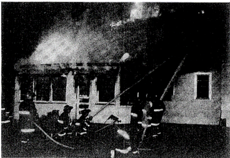
ARSON FIRE, RIVER ROAD - 1975
